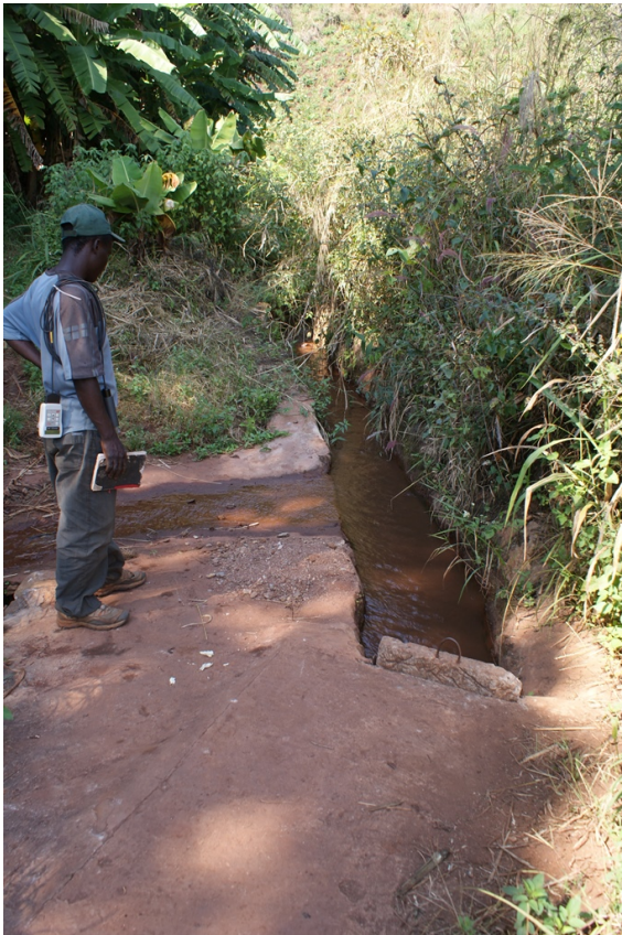
Figure A.55: One of the headwaters of Chirodzo (location Chir_1_1_us_in), the stream is regulated with a (leak) valve (bottom of the picture), from which water continuously flows in the Chirodzo stream. The side spill flows into an irrigation canal. Holsteijn [10] took here his measurements (June 2014)
