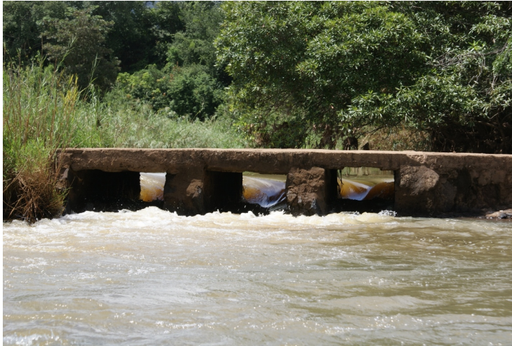
(a) Gates Messica bridge
