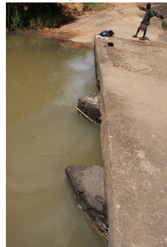
Figure E24: Opening bridge gates, observe the orientation angle of 27^\circ
