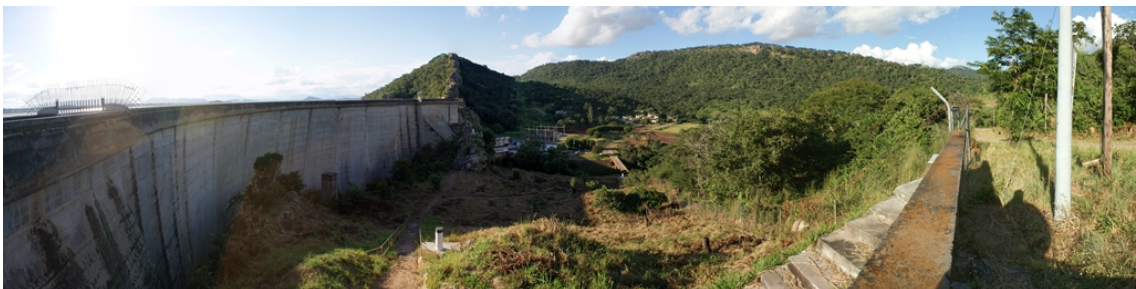
Figure A.37: Chicamba dam. (March 2014)
