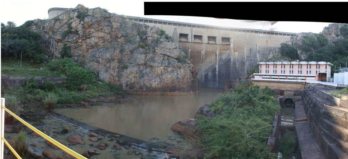
Figure A.39: Chicamba Dam (March 2014)
