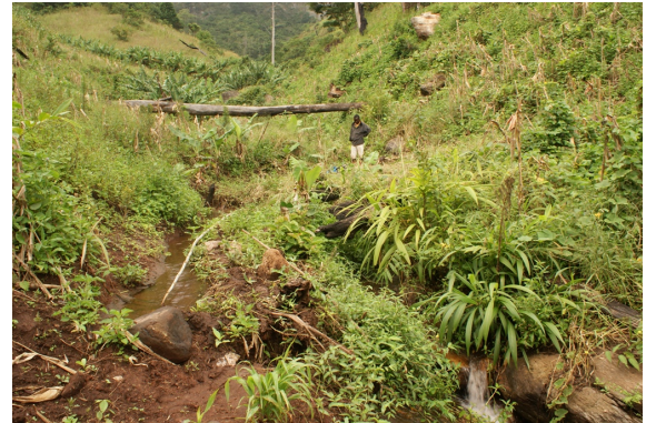
Figure A.54: Start of an irrigation canal in the Godi Catchment (Location Godi_1_1_us_in). At the right side, the Godi stream continues, at the left side the irrigation canal, which ends up in a pipe to bridge a steep slope Fig. A.56. (April 2014)
