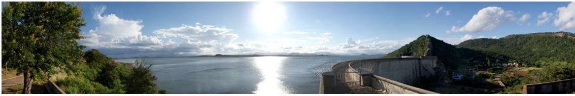
Figure A.38: Chicamba Dam (March 2014)
