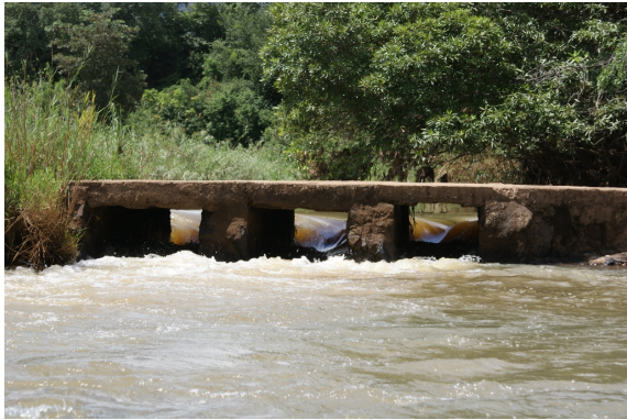
Figure E21: Free-flow (spillway) bridge Messica downstream
