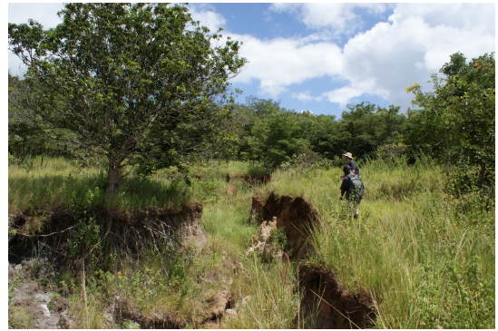
Figure A.46: Gully in Ruaga Catchment. Observe greyish soil, at the left side and red coloured soil at the left side of the gully. The gully increases during rainseason 2013-2014 from the tree at to the end, a length of about 30m. (March 2014)
