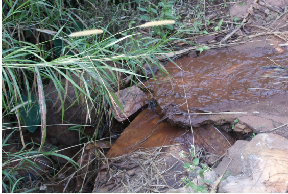
Figure A.53: Downstream outflow at Chirodzo from Fig. A.55 (where the valve is completely closed) (June 2014)
