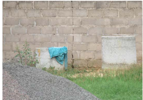
Figure 8.24 Groundwater borehole well as future alternative (not operated yet)
