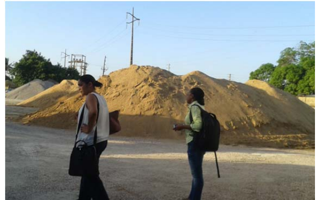
Figure 8.15 The open storage of aggregates
