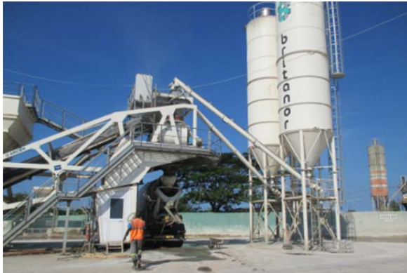
Figure 8.27 The clinkers with a truck beneath it being filled-up with ready-mix concrete
