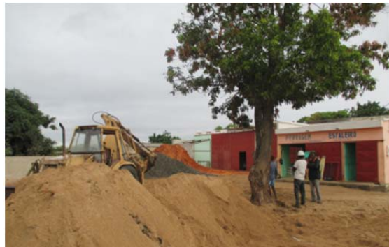
Figure 8.3 Preparation of a house construction
