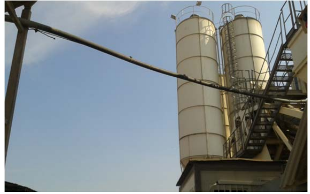
Figure 8.20 The clinkers and the horizontal hose (The hose brings the effluent of decantation system is used again in the concrete mixture)
