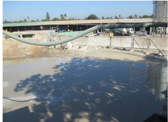
Figure 8.34 Decantation pond (for water recycling system)
