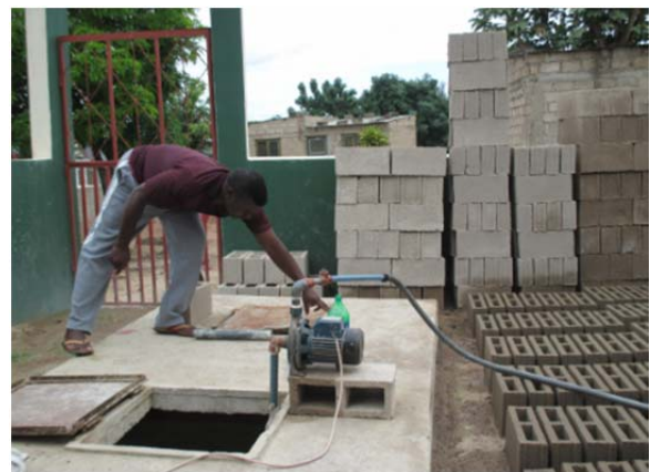
Figure 8.10 Pumping water out of the decantation tank to be used for curing again
