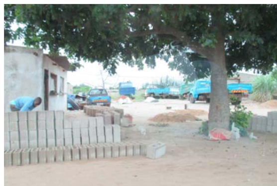
Figure 8.4 Concrete blocks for the walls
