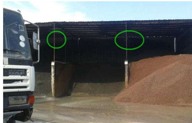
Figure 8.18 The aggregates are being sprinkled with water (The sprinklers are circled)
