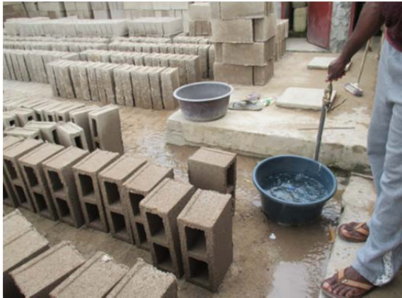
Figure 8.7 Curing the concrete blocks (The floor has a slope to collect water into a small side ditch)
