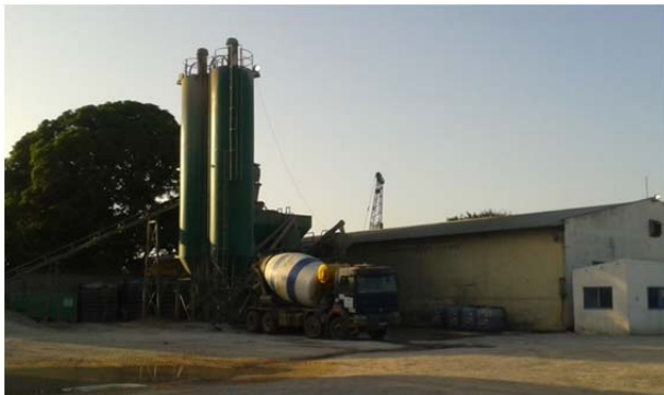
Figure 8.14 The clinkers and truck ready to be filled-up
