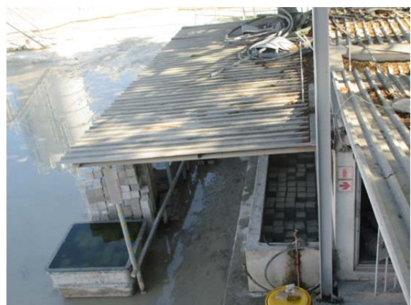
Figure 8.35 Curing pond
