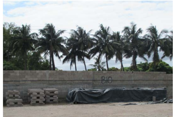
Figure 8.25 Curing with fabric cover to reduce water consumption
