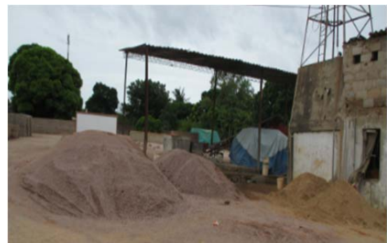
Figure 8.12 Storage of bulk materials
