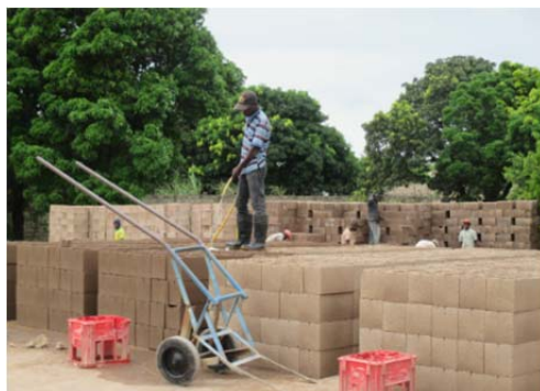
Figure 8.11 Curing by sprinkling with flexible hose
