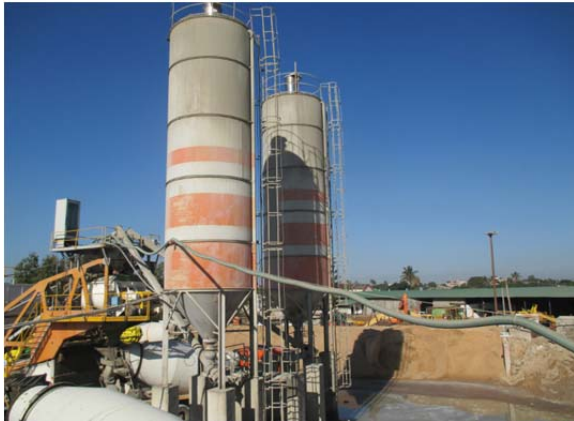
Figure 8.32 The clinkers and a hose that supplies water
