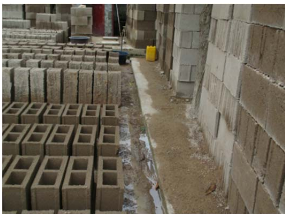
Figure 8.8 Small ditch traps the excess of curing water and transports it to the drain
