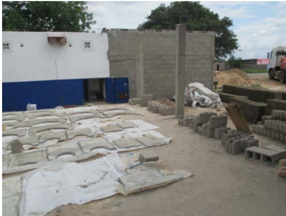
Figure 8.1 Freshly-hardened latrines
