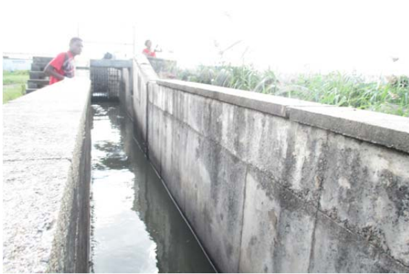
Figure 8.43 Influent from the main sewer
