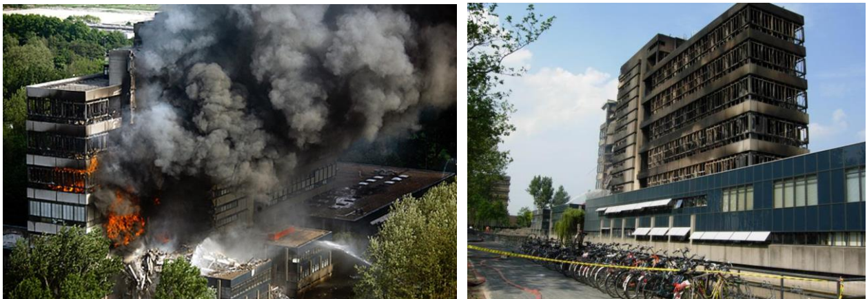
Figure 1: The Faculty of Architecture building being on fire and after the fire
