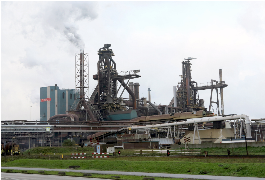
Figure 23: Blast Furnace 6 (left) and Blast Furnace 7 (right), which is going to be decommissioned first during the transition phase at the site of Tata Steel in IJmuiden, the Netherlands. Combined they can produce more than 650 tons of Hot Iron per hour.
