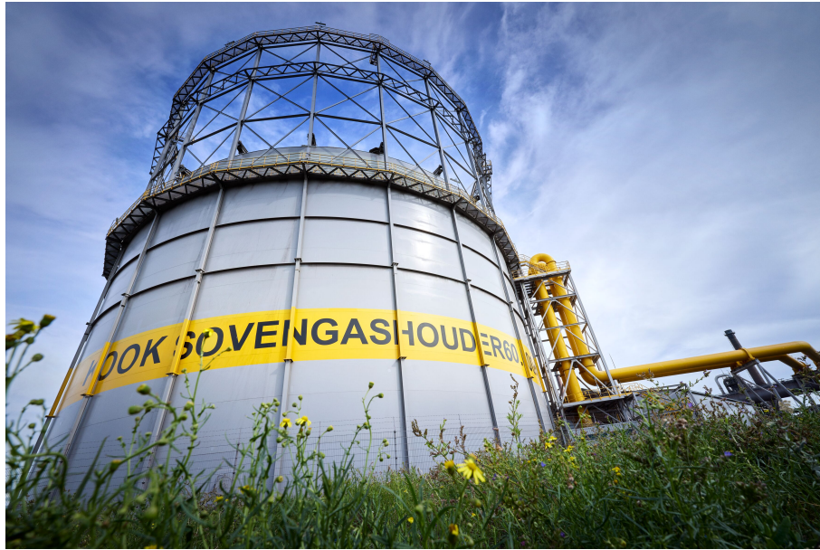
Figure 37: One of the Gas Holders of the site in IJmuiden that is used as a buffer for short-time storage of Coke Oven Gas
