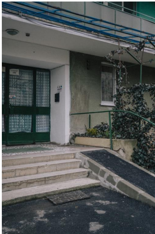
Figure 4: Nistor, Cristina. 2024. Entrance of block, handrail and ramp only recently added. Photograph taken by the author.
