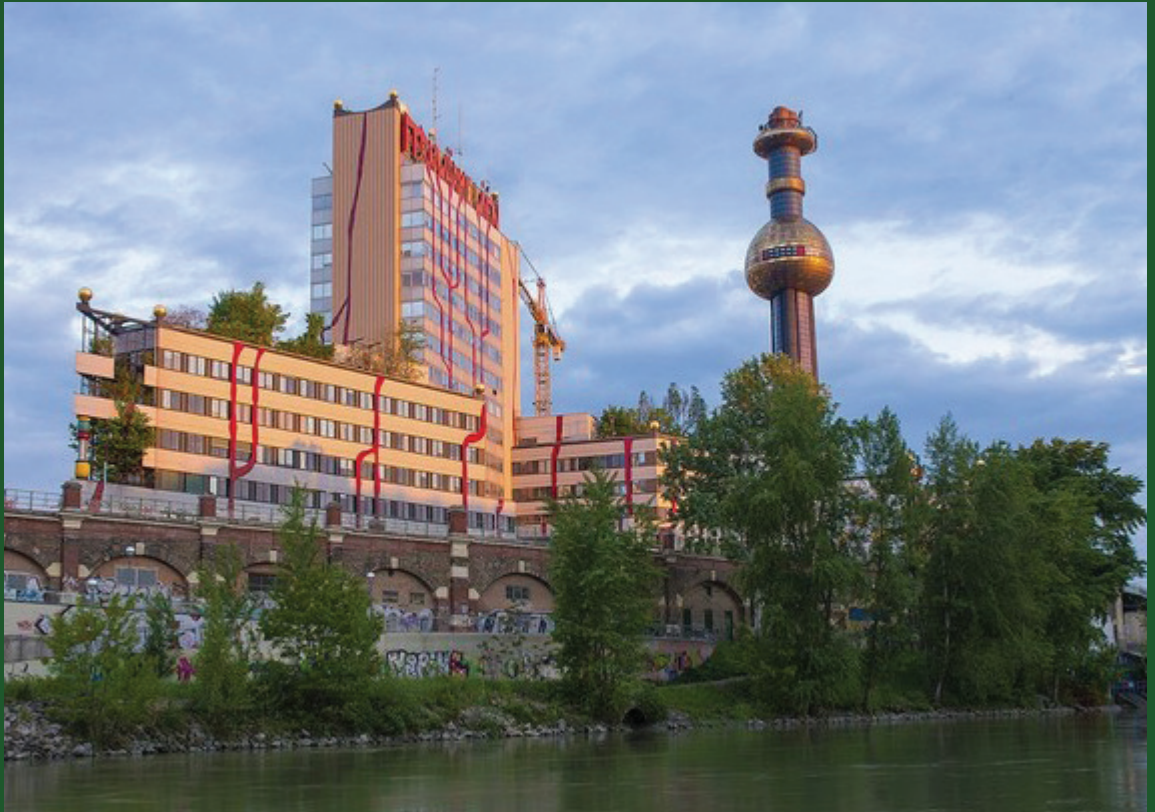
Spittelau waste plant from river. ®
