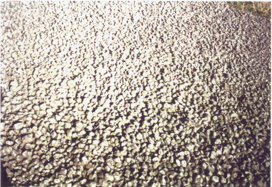
Fixtone open stone asphalt placed on sand asphalt on sand Hartel Canal
