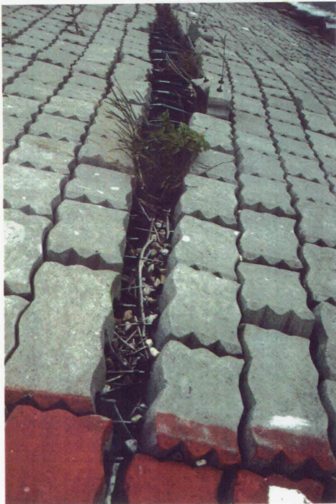
Picture 10: Beto-mat; detail of the internal joint between standard mat sections
