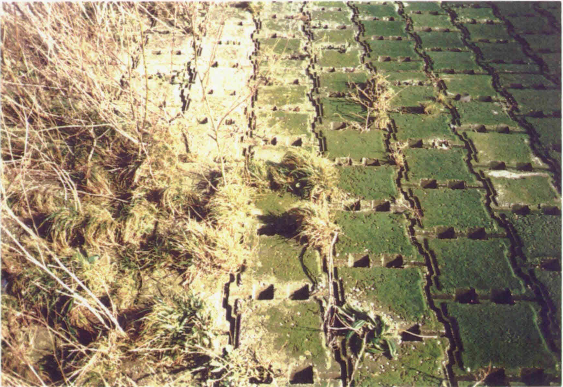
Armorflex block mats placed on gravel (Hartel Canal)
