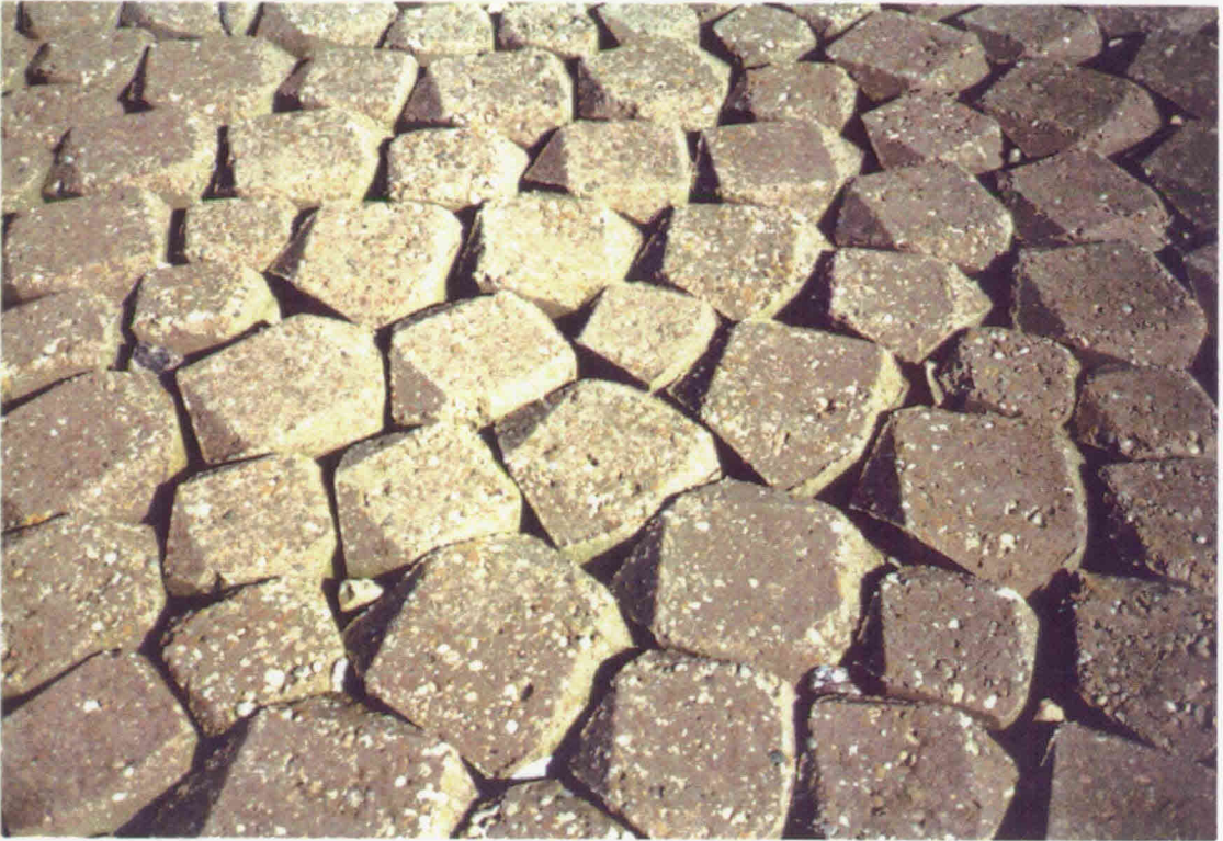
Basalt blocks placed on silex and on geotextile/sand (Hartel Canal)
