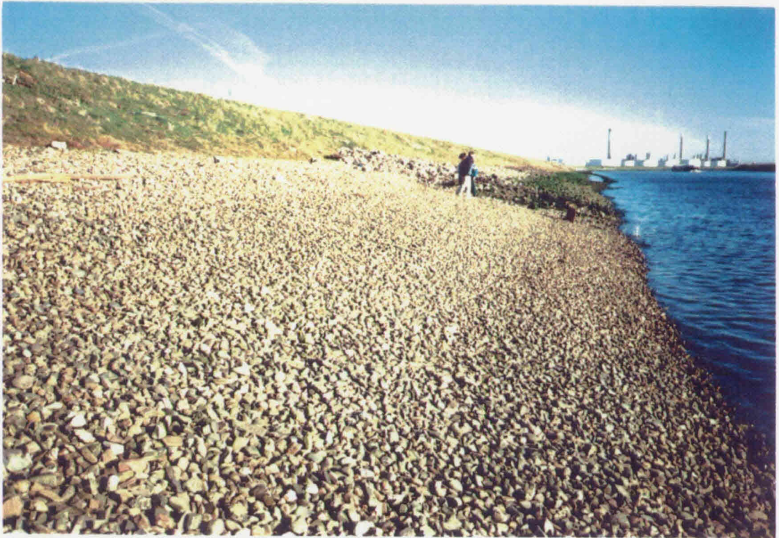
fine gravel (30-80 mm) on geotextile on sand (Hartel Canal)
