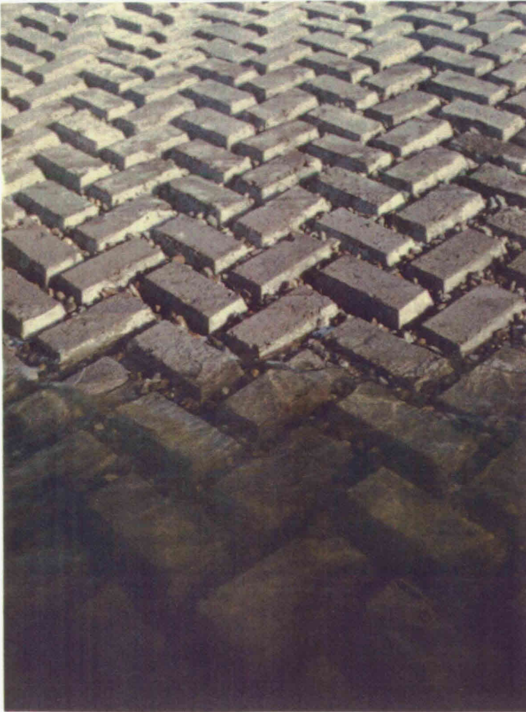
ACZ-Delta block mats placed on geotextile/ gravel (Hartel Canal)
