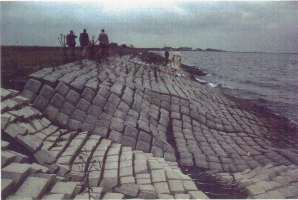
Picture 3 : V.O.B./ASAM; transition between both mat types
