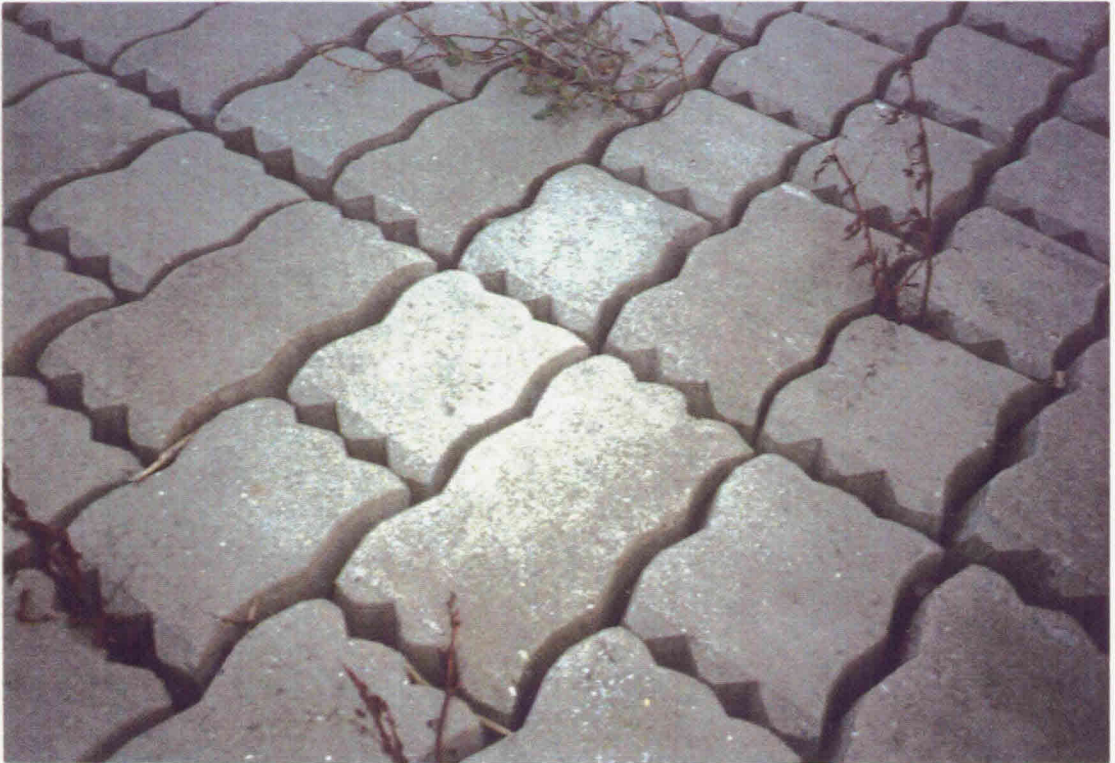
Beto-mat placed on a geotextile on minestone and on sand (Houtrib-dike), showing joint between 2 adjacent sections
