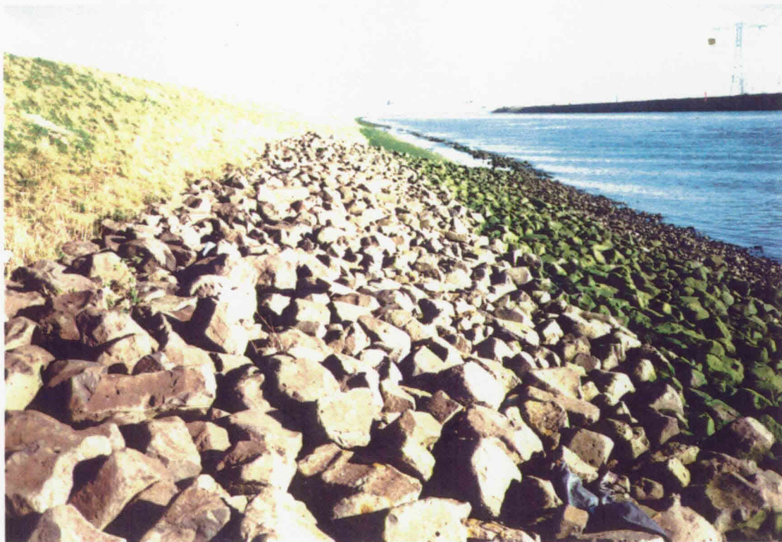
rip-rap (5-40 kg) on geotextile, both on clay and on sand (Hartel Canal)
