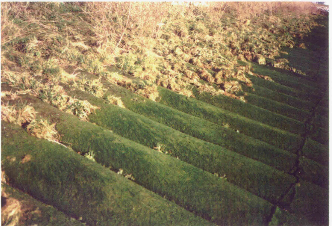
sand-sausage mattress Profix placed on gravel (Hartel Canal)
