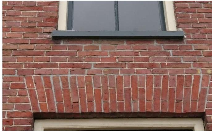
*Figure 4: A repaired masonry wall*
