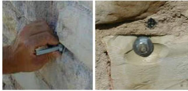
Figure 12: Positioning of stainless-steel threaded bars as ties
