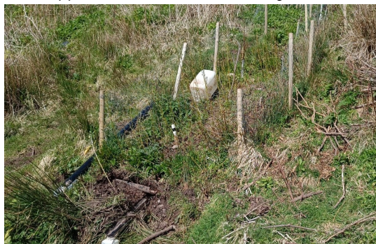
(e) Live pole drain, located at D in Figure 5.3
