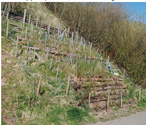
(g) Cribwall, located at C in Figure 5.3
