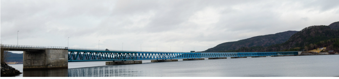
Figure 1: The Bergsøysund Bridge. Photograph: K.A. Kvåle.
