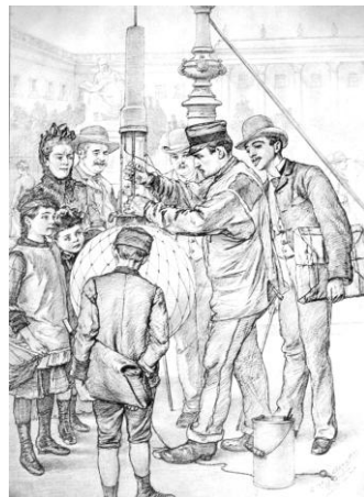
Figure 55: Replacement of electrodes (Berlin, 1889).
