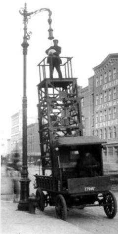
Figure 56: Maintenance of arc lamps (ca. 1890).
