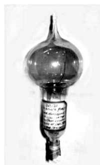
Figure 86: An Edison bulb that was used to light his Menlo Park laboratory (1879).
