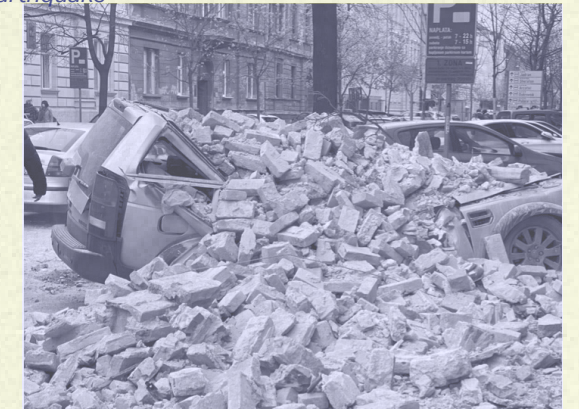
Figure 18. - damaged outer walls of historic buildings, fallen on nearby cars in the city centre
