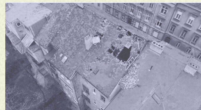
Figure 21. - damaged roofs due to old chimneys falling through
