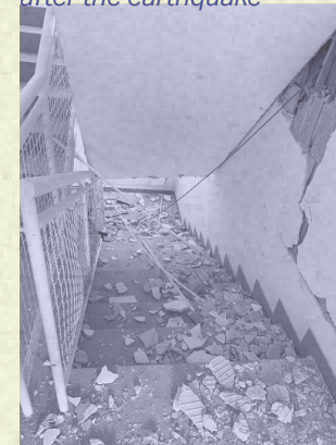
Figure 16. - damages to an improperly built building in ZG
