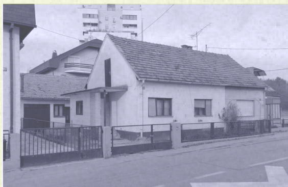
Figure 12. - private masonry house, without reinforcement
