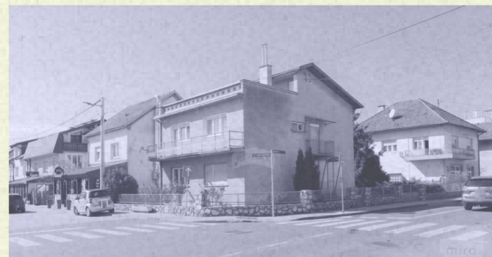
Figure 13. - private masonry house with little to no reinforcement
