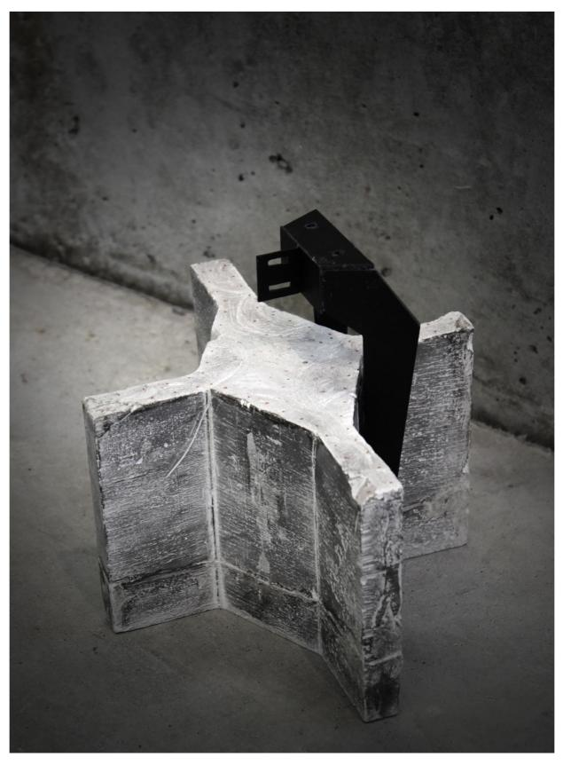
2. placement first part claw, chemical anchoring to concrete
