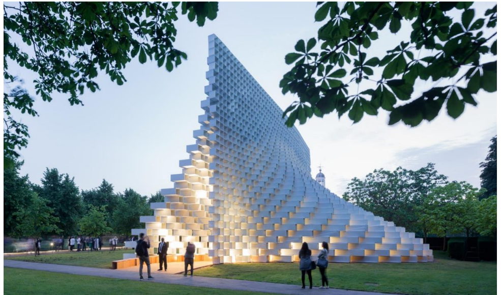
Figure 77. Serpentine Gallery Pavilion by BIG, London, UK, 2016. Constructed using GFRP boxes (source: dezeen.com)
