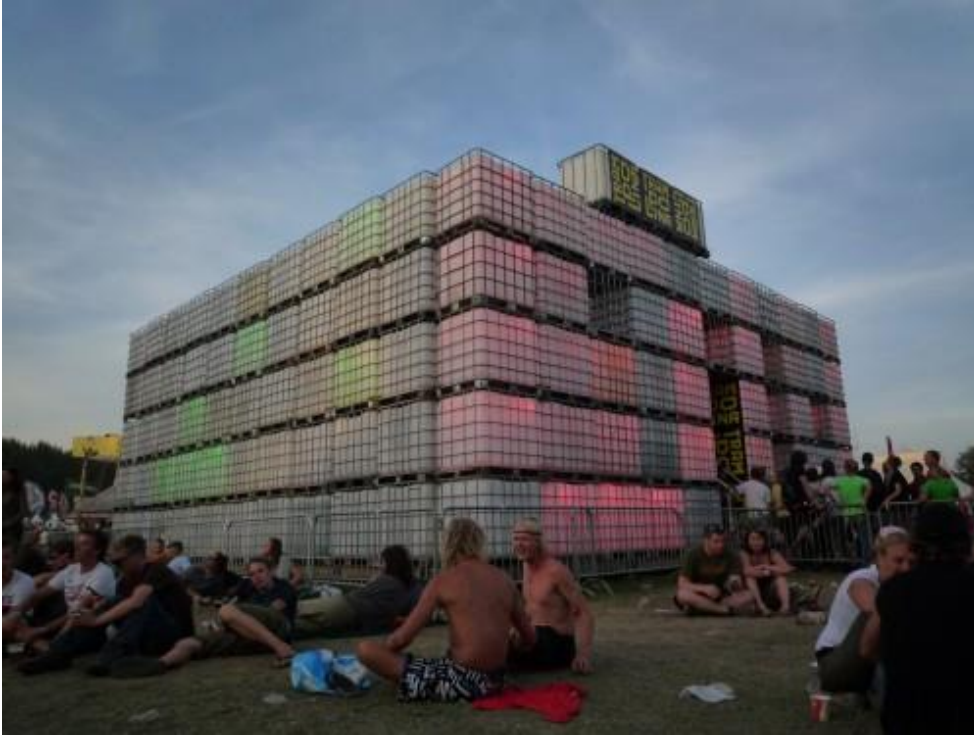
Figure 78. Recropolis by Refunc studio, Biddinghuizen, Netherlands, 2009. Structure constructed from 240 reused water tanks (source: refunc.nl)
