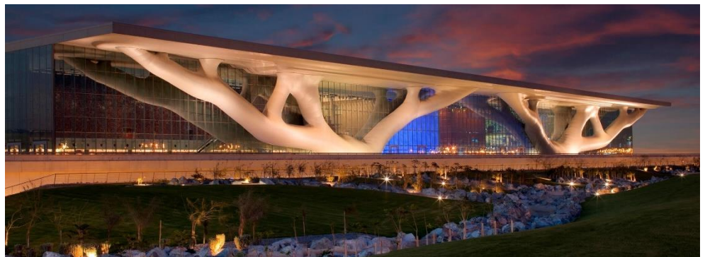
Figure 36. QNCC exterior part of the topologically optimized columns (source: http://archdaily.com )
