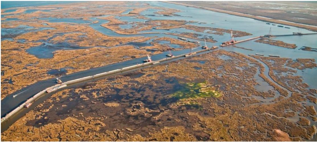
**Figure 2-25: Construction of the Inner Harbour Navigation Channel/St. Bernard storm surge barrier (photo Royal Haskoning)**
