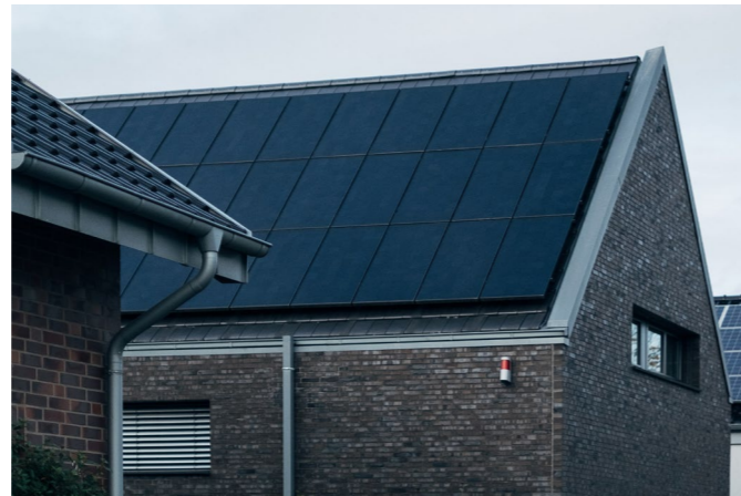
Figure 15 A sustainable house with solar panels
