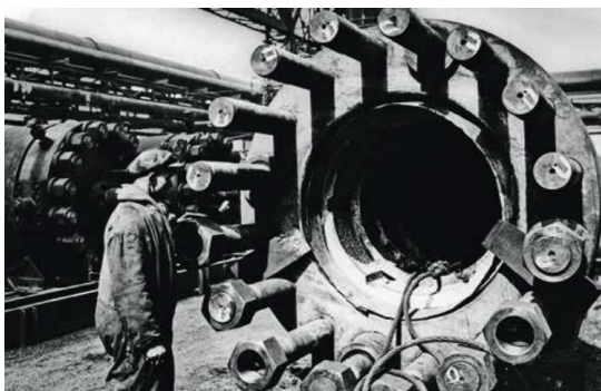
Figure 2.1: An example of a BASF high pressure reactor from the 1920's. Although it cannot be stated with certainty this specific one is a methanol or ammonia reactor they were highly alike. Figure adapted from [28].
