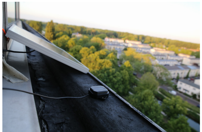
N.2. Solar panel and U-blox antenna at South-east side of building
