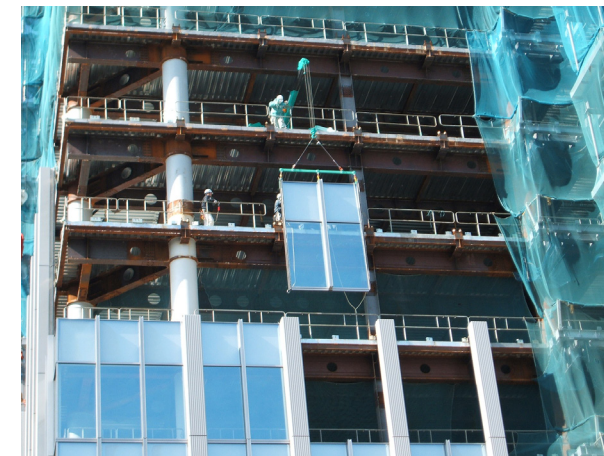
Figure 2.2.1: Curtain wall assembly during construction (Source - https://www.maedausa.com/mini-crane/mc285-2-curtain-wall-installation-13433570753-o/ )
