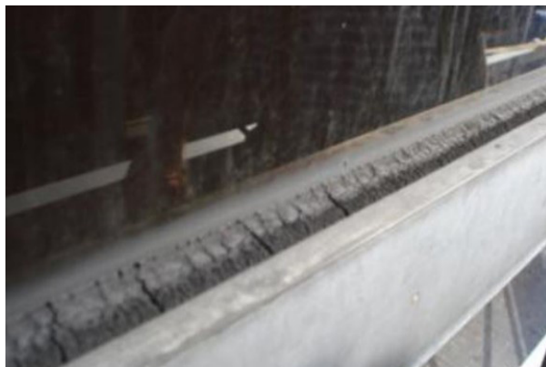
Image 3: Dried and damaged gaskets
