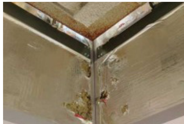
Image 4: Damaged vapor barrier
