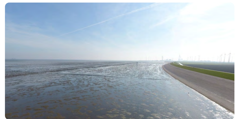
Figure 1: Dike partially covered by asphalt and partially by grass, fronted by a shallow, mildly-sloping mudflat along the Dutch Wadden Sea coast. Photo by Jaap van Duin.
