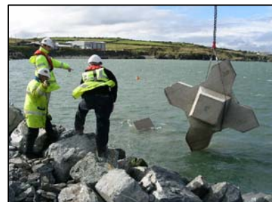
Figure 5.3 Xbloc Unit in Port Oriel
