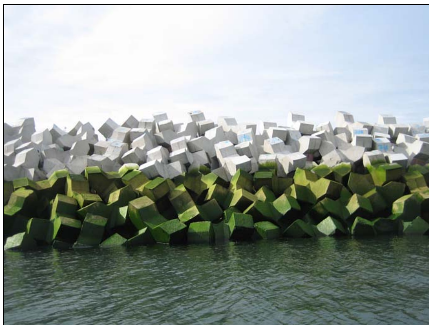
Figure 5.6 Xbloc Unit on the Trunk Section of the Port Oriel Breakwater
