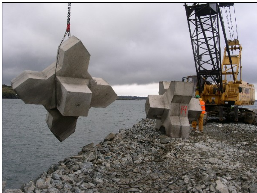
Figure 2.7 Xbloc Prototype unit attached to a sling Lifted by a Crawler Crane
