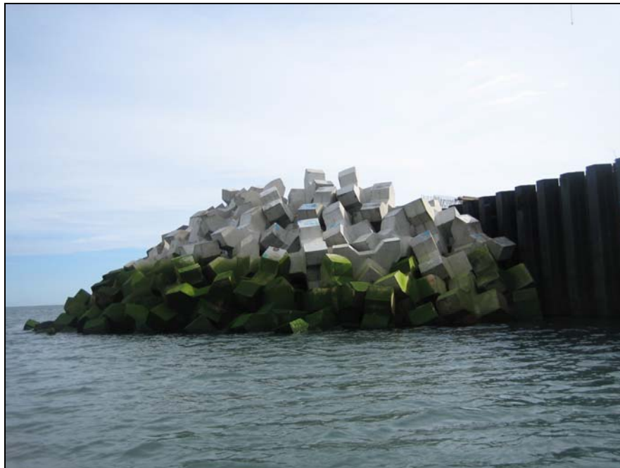
Figure 5.7 Xbloc Units on the Head Section of the Port Oriel Breakwater
