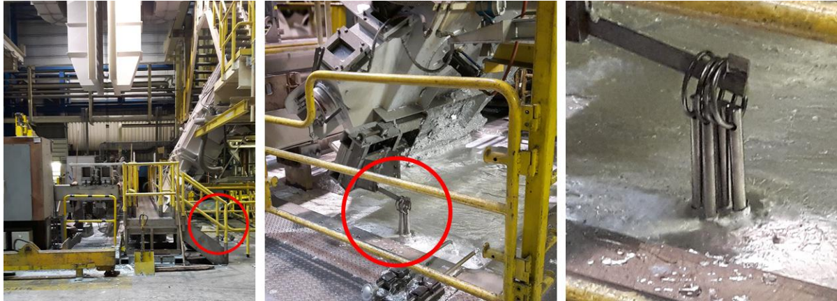
Figure 4-1: Photos of where the sample rods are positioned in the Zn-bath in DVL 2. A schematic representation is shown in Figure 4-3
