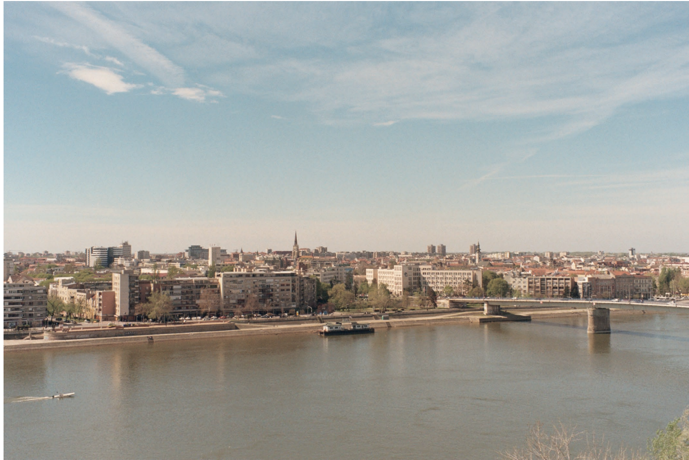
The Danube at Novi Sad with the Varadin bridge.
