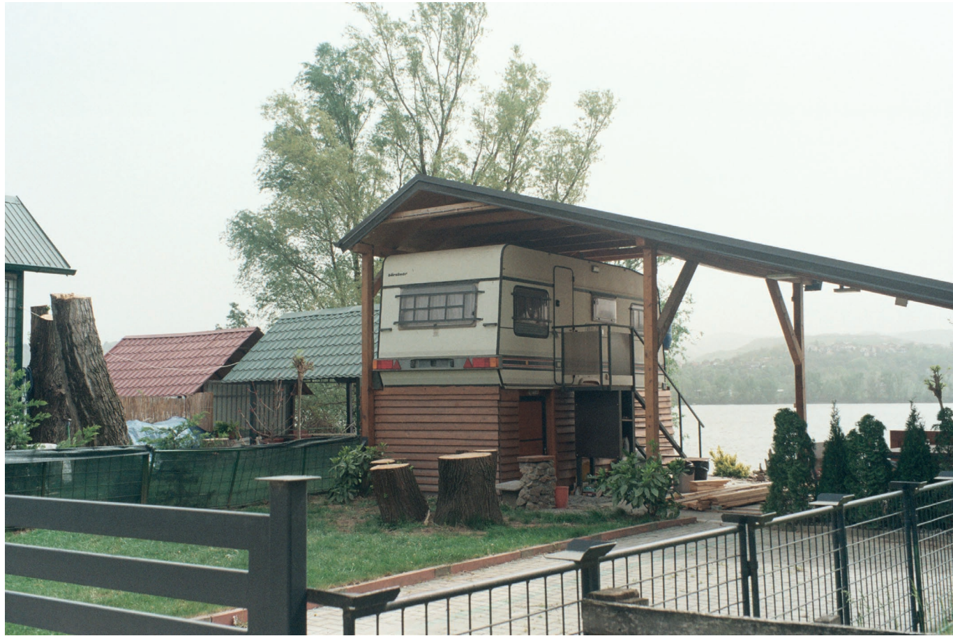
Adapatation to the fluctuation of water levels on one of Kamenička ada's illegal houses.
