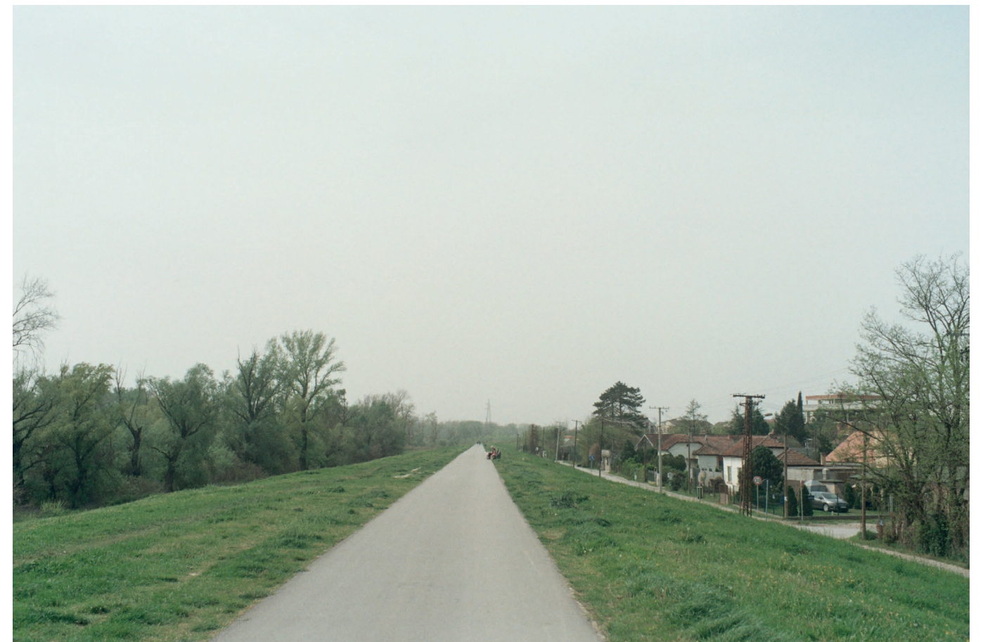
The protective embankment of Novi Sad along Kamenička ada, seen on the left of the image.
