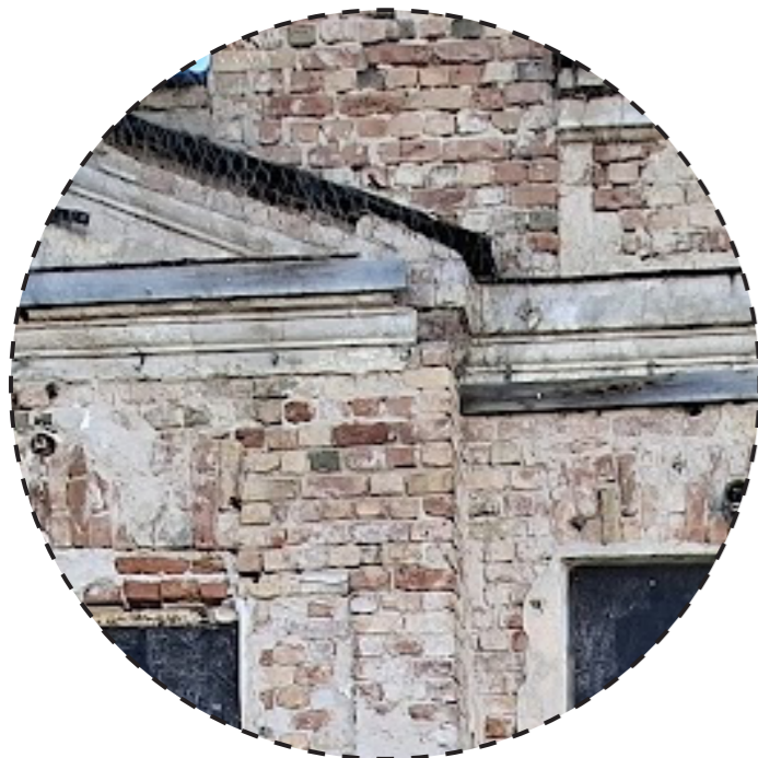
EXISTING WALL (SANDED)
