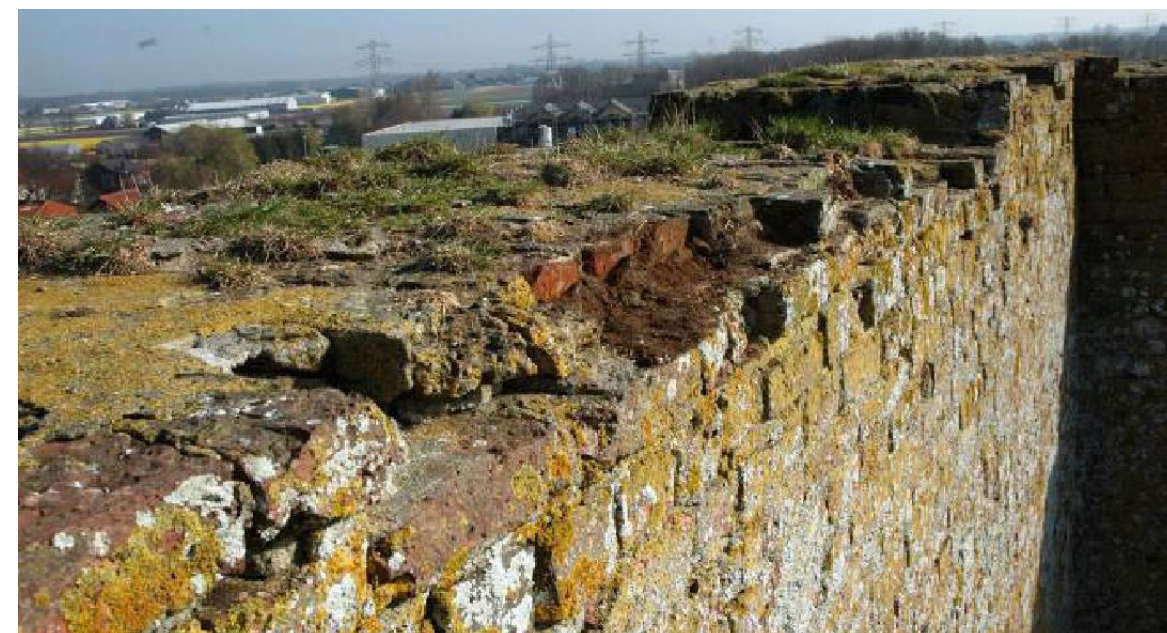
Damaged top surface walls -> uneven
