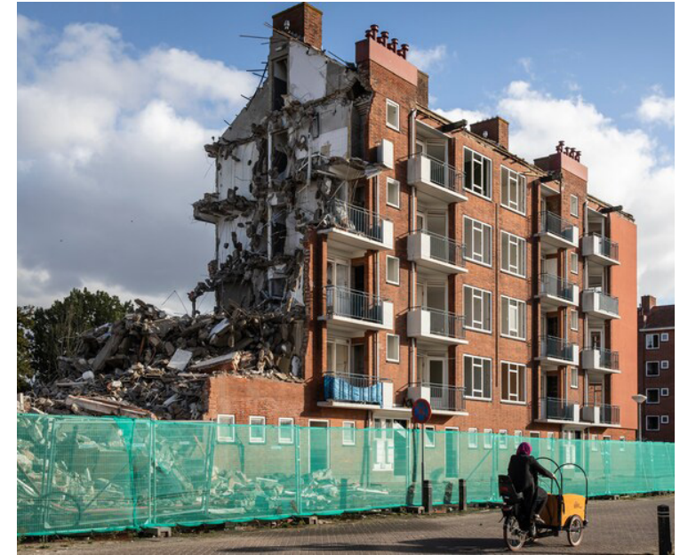
Picture 1: demolition in Amsterdam Nieuw West
