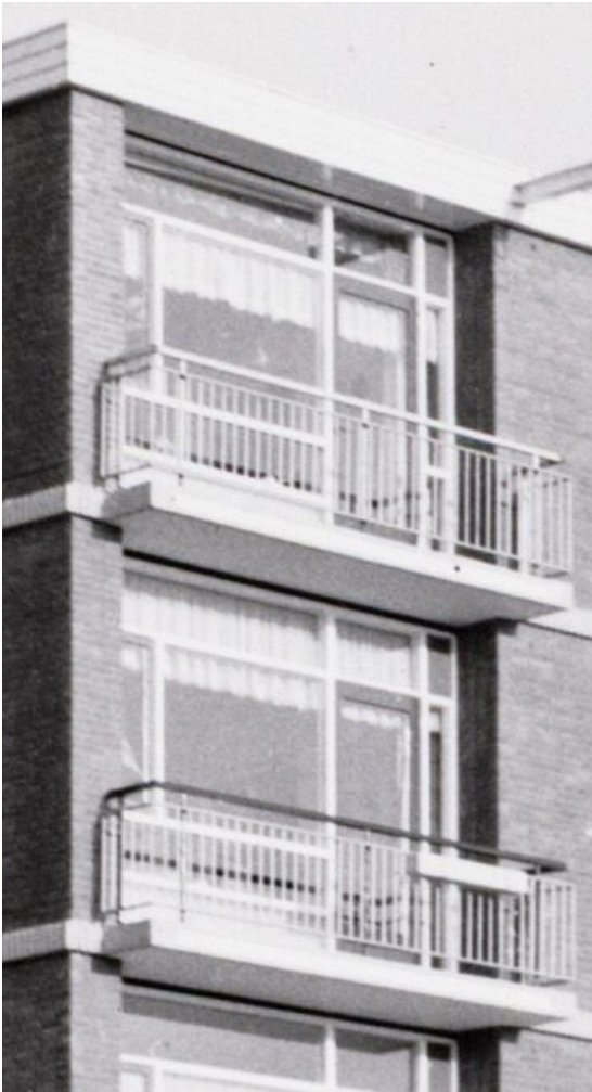
Picture 5: historical photograph of facade fragment. Seen in the picture are the storey-high windowframes that lead to the balcony.
