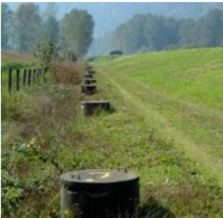
Figure 3.4: Relief wells system. Source: [City of Chilliwack,2008].
