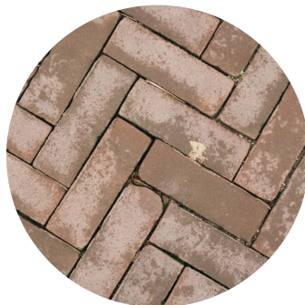
Figure 7. Water-passing pavement 7
