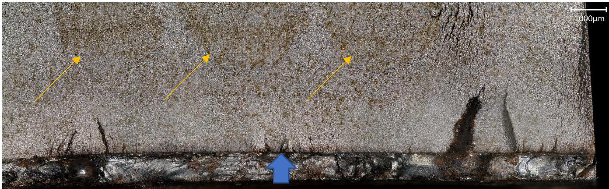
Figure I. Zoom-in view of the specimen Ex-A, presenting the arch-like features along the weld root. Crack growth direction marked with the blue arrow.
