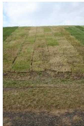
Figure 3-4: After placing the Geogrid (left), the test section was covered again with the grass from big rolls (right)
