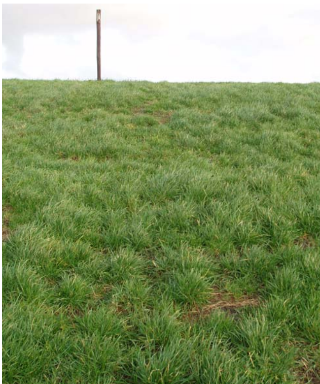
Figure 3-5: Impression of the SGR test section prior to testing (winter 2006-2007)
