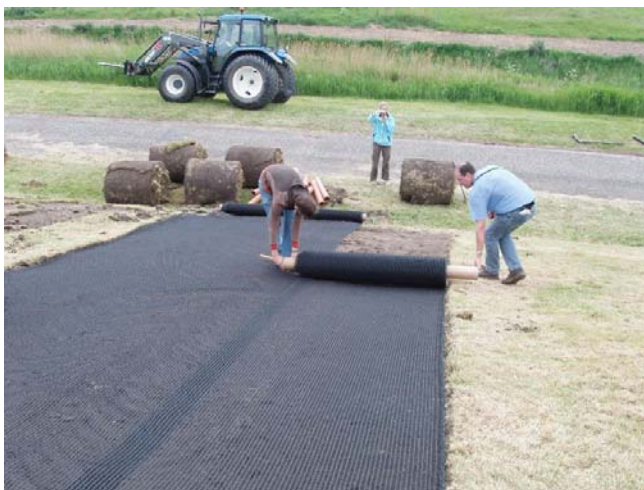
Figure 3-4: After placing the Geogrid (left), the test section was covered again with the grass from big rolls (right)
