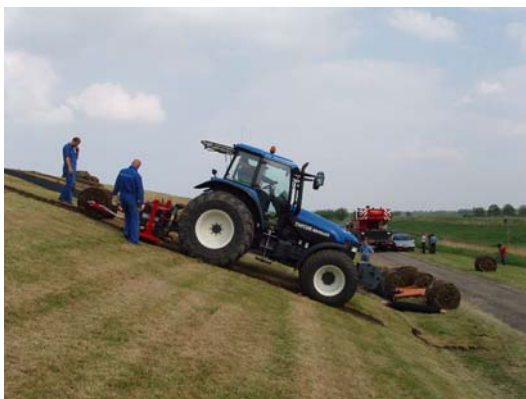
Figure 3-3: Finally selected methodology: cutting in downward direction
