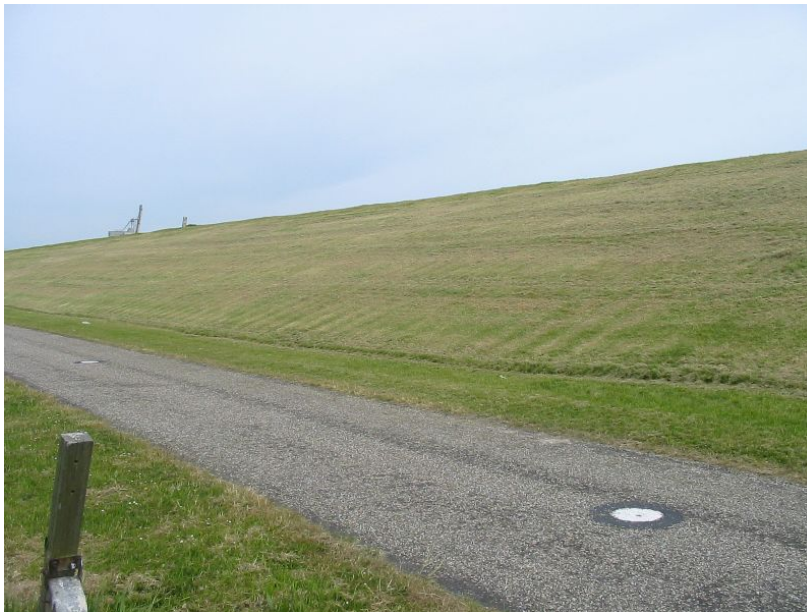
Figure 5-2: Overview of test section location before placement of the SGR (spring 2006)
