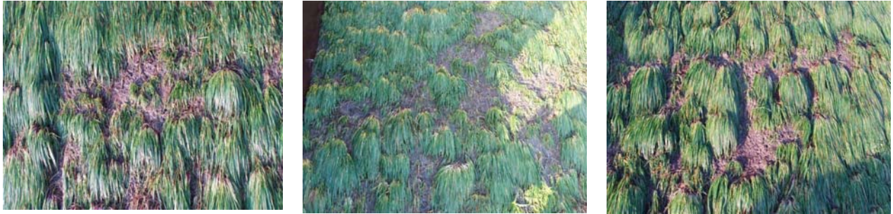
Figure 10-2: Detailed photographs of some bare spots after the 10 l/s/m test at the reinforced test section
