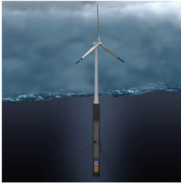
Figure 1.3: Spar Floating wind turbine: Hywind prototype Statoil Hydro. Image property of Siemens, taken from NS energy publication [66]
