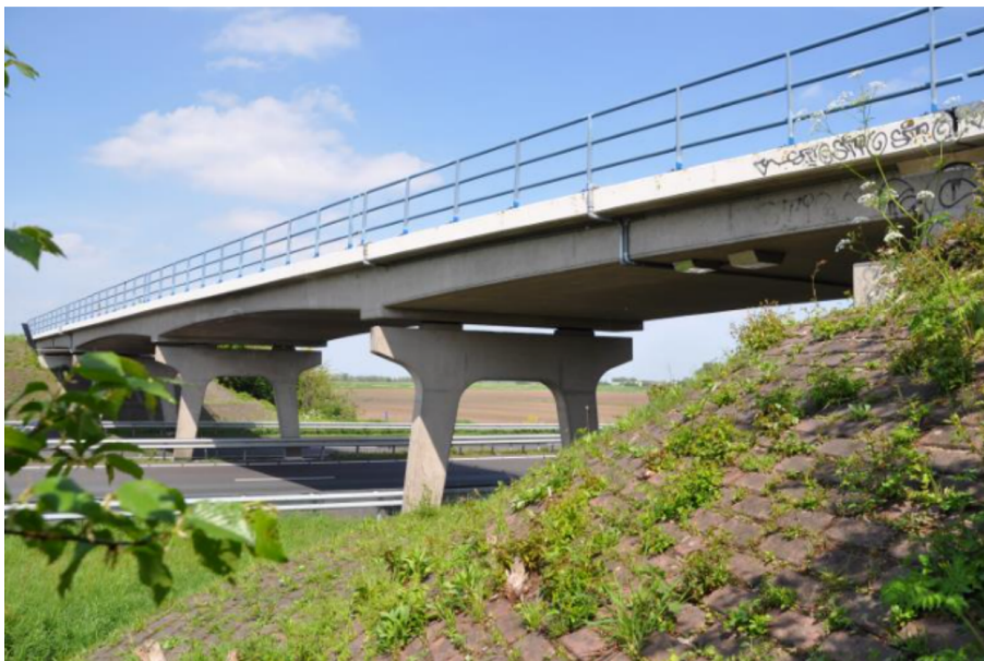
Figure 3.1: Typical slab bridge [12]
