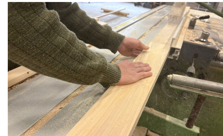
Figure 4: Planing fingerjointed and laminated poplar beams
