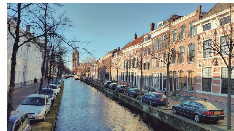
Figure 13. High quays without vegetation for human safety and a neat streetscape lead to drowning hazards for hedgehogs, frogs and young swans, among others.
