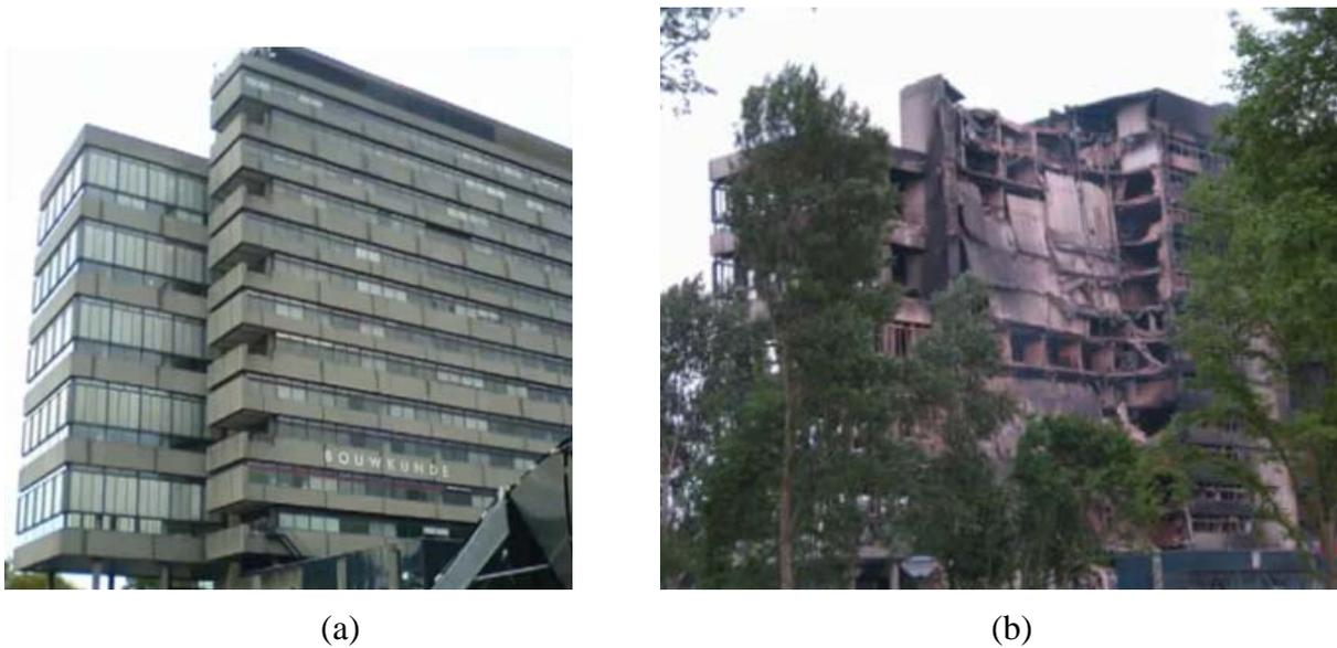
Fig. 1.2 Architecture building before (a) and after (b) fire in Delft University of Technology.
