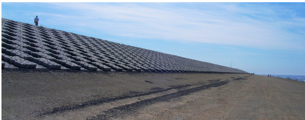
Figure 3.1 Roughened outer slope of the Hondsbossche Sea Defences by introducing different height of the concrete elements
