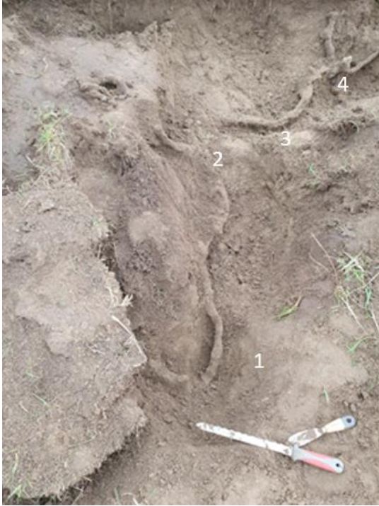
Figure B1: Overview of excavated tunnel, numbers indicate location of detailed images
