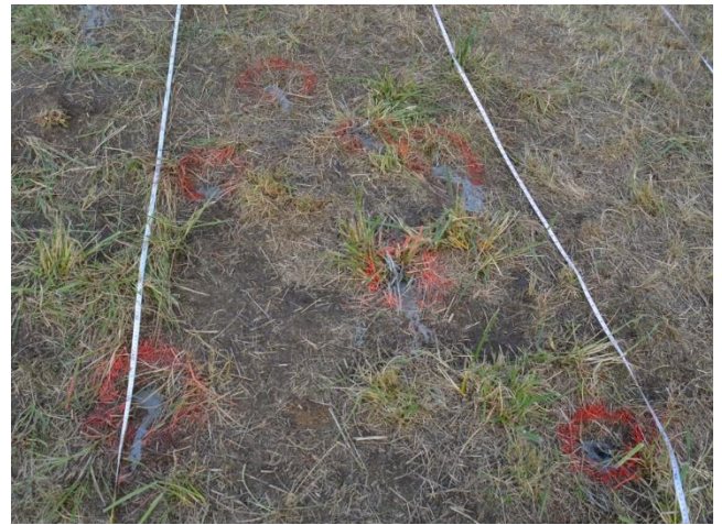
Figure 12: Numerous grout-filled burrow holes on the coordinate grid
