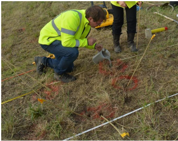
Figure 11: Filling a burrow hole with grout
