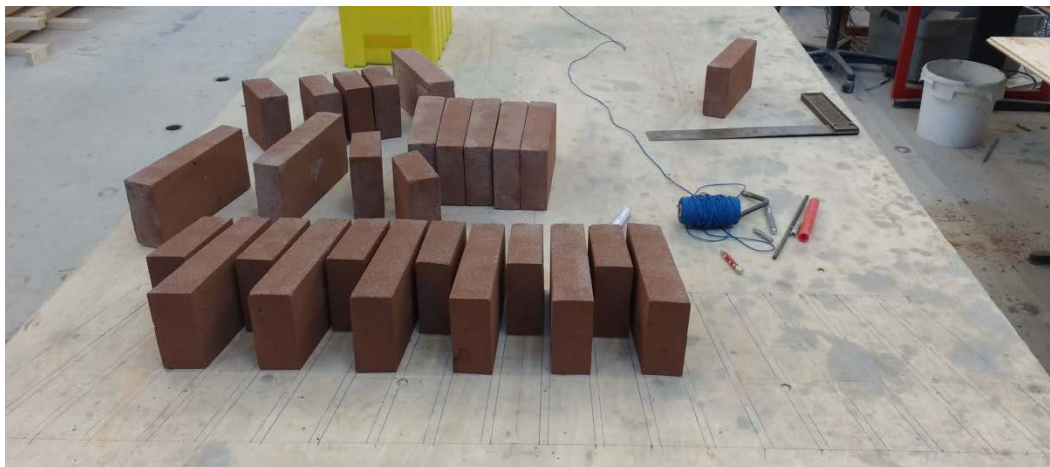
Figure 45 – Cutting template for jack arch
