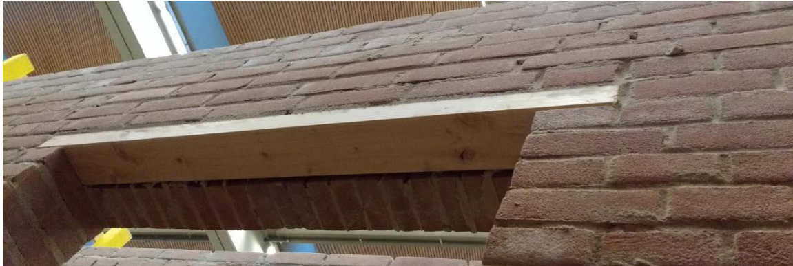
Figure 44 - Wooden beam to support masonry above window opening
