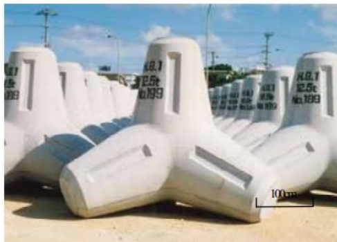
Figure D.15: Armour units made of concrete, with gutters on surface (Akakura, 2005).
