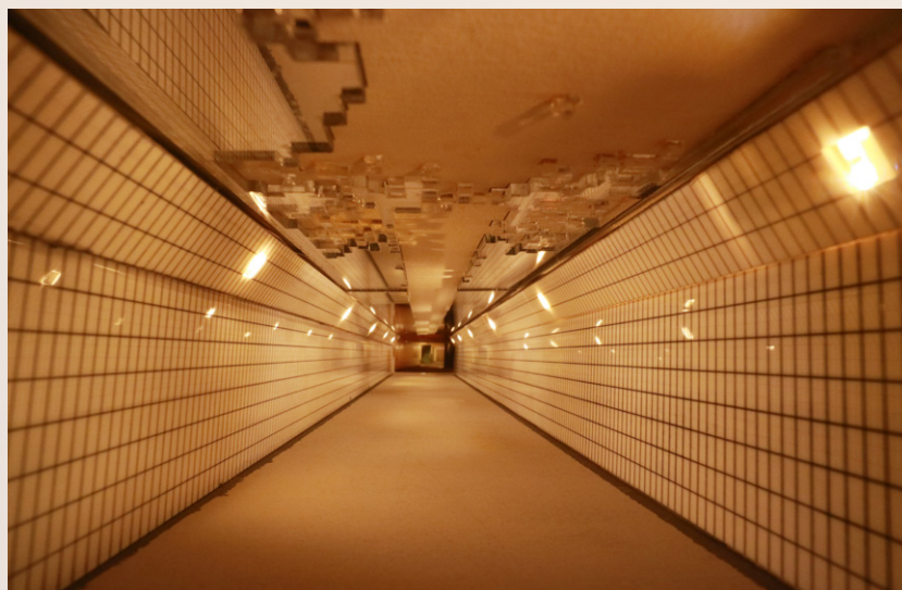
Figure 6.4 The photograph of the design using mirrors to decorate the Maastunnel presented in a 1:40 scale model. Although the dummies are not shown, they are present in the evaluation session as a relative size visual cue.
