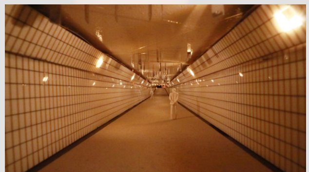
Figure 5.3 Photos of hanging spangles in the tunnel (a) without the roof and the lighting on and (b) with full installation of the tunnel. The size of a spangel is about 3 mm x 10 m.
