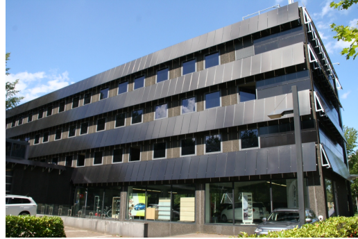
Figure 15: Thin film façade panels on an office building in Amstelveen, the Netherlands.
