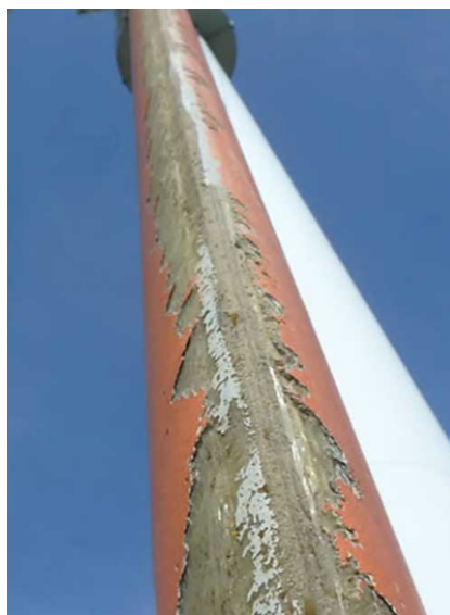
Figure 2.1: Leading edge erosion of wind turbine blades [19].
