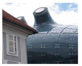
Left: view of Kunsthaus Graz in the middle of Graz, Austria. A 'Friendly Alien' in a historical setting. right: close-up of a 'Nozzle'; cladding was done in PMMA panes with point fixations..
