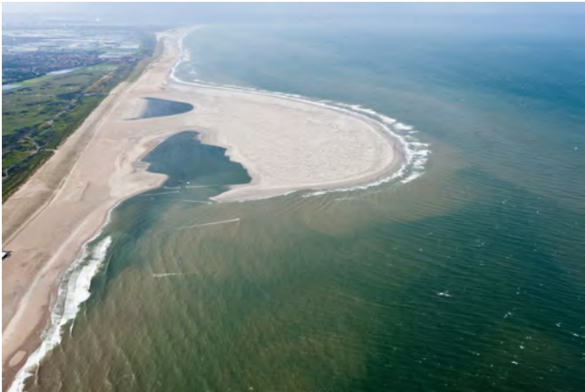
Figure A-1: The Sand Engine in September 2011 (Photo from: flickr.com/photos/zandmotor)
