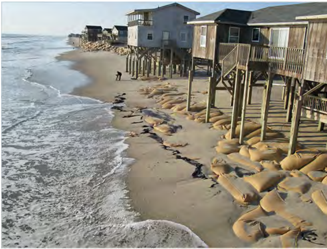
Figure 1-1: Example of an erosion problem which is a combination of shoreline retreat and human functions that are at risk (Source: Barringer)
