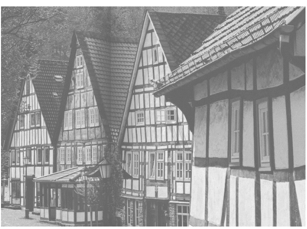
Fig. 29: traditional German half-timbered house. The timber skeleton carries the weight of the light earth infills. The infills are a mixture that contain high amounts of straw and other fibres to reduce the weight and increase the insulation properties. Source [6]
