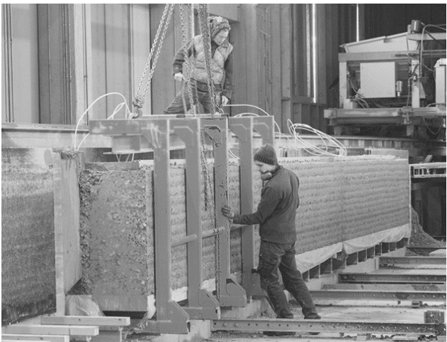
Fig. 34: Assembly of a prefab, monolithic rammed earth wall. Schlins, Austria, 2019. Source: [21]
