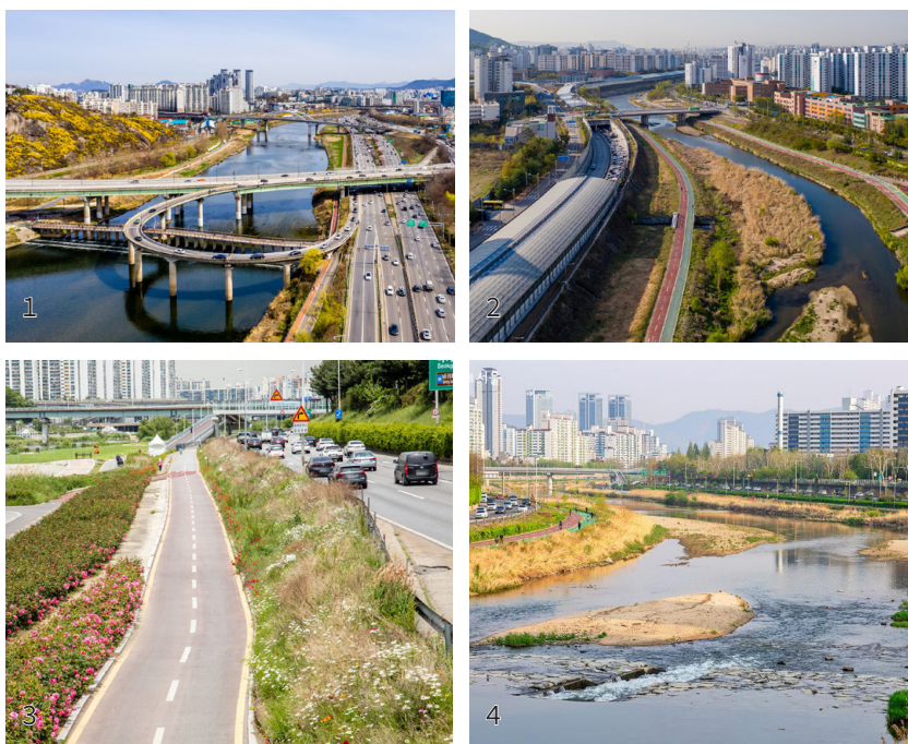
Figure 58 : Relationships with adjacent infrastructures in Jungrang stream
