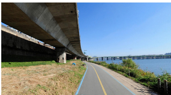
Example of river promenades between parks: Promenade between Hangang-4N and Hangang - 5N
