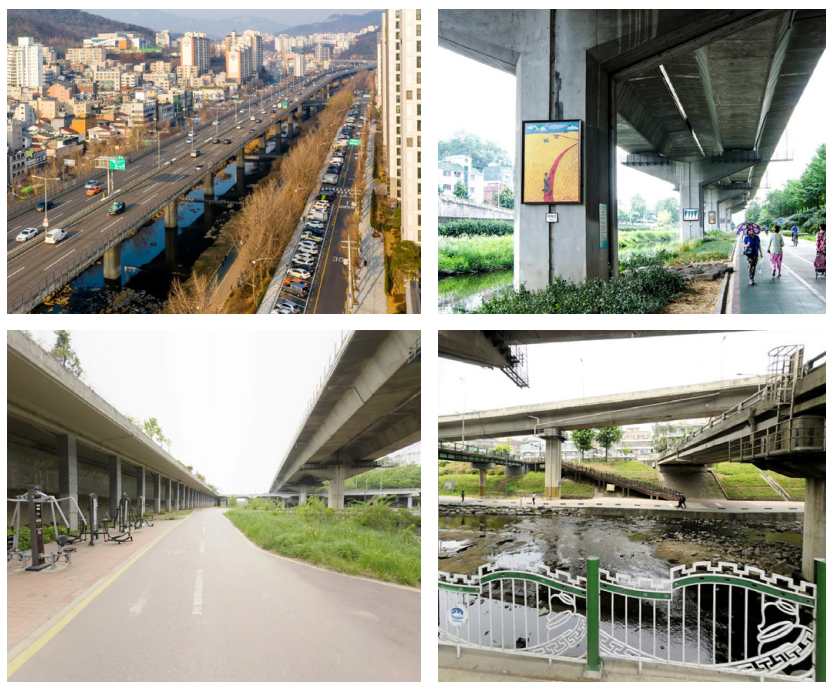
Figure 85 : Relationships with adjacent infrastructures in Hongje stream
