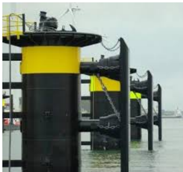
Figure 1.1: Typical flexible dolphin in the Port of Rotterdam. [5]
