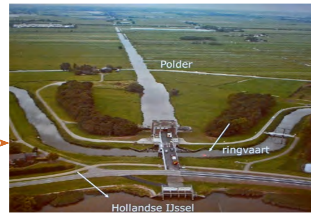
Fig. 47. The Abraham Kroes pumping station. ( https://www.diegoude.nl/wp-content/uploads/2019/08/Lezing-2019-05-27.pdf ).
