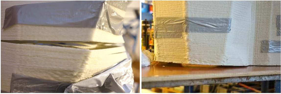
Figure 7.21: Cracks caused by shrinkage. Left: large crack at outer surface. Right: Warping of the bottom of the mould.
