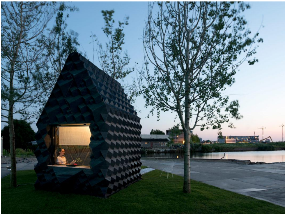
Figure 1.1: 3D printed Urban Cabin by DUS architects [3] (photo by Ossip van Duivenbode ).
