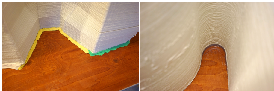
Figure 7.13: Bottom sealing. Left: clay at outside. Right: Silicon at inside.
