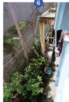
A house condition after joining the renovation project
